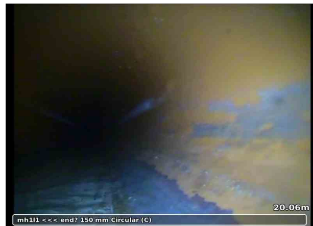
4, 20.00 m Settled deposits, coarse, 20% cross-sectional area loss
