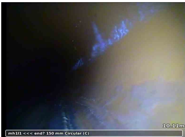
3, 10.00 m Settled deposits, coarse, 20% cross-sectional area loss
