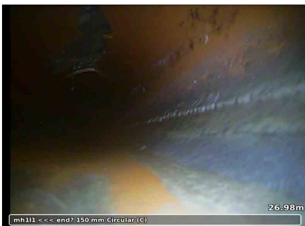
5, 26.98 m Fractures, multiple from 12 o'clock to 12 o'clock
