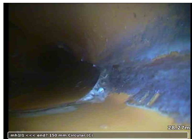
6, 28.27 m Fractures, multiple from 12 o'clock to 12 o'clock
