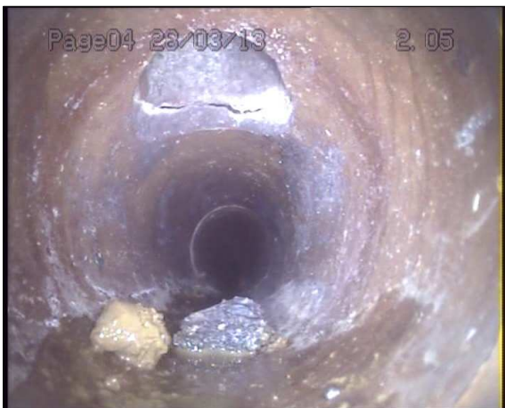
Photo: 1_1_6_A.jpg 2.1m, Connection, at 12 o'clock, 100mm diameter
