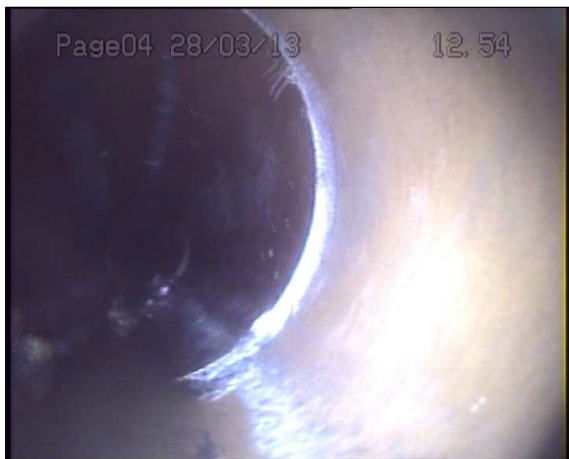
Photo: 1_1_20_A.jpg 12.7m, Joint displaced, medium (between 1.0 and 1.5 times the pipe wall thickness)
