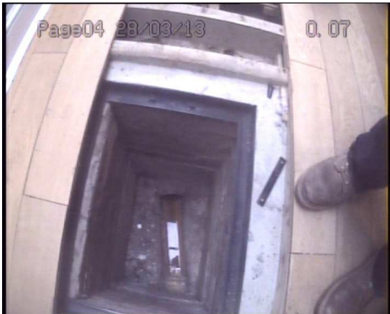
Photo: 1_1_1_A.jpg 0m, Start of survey
