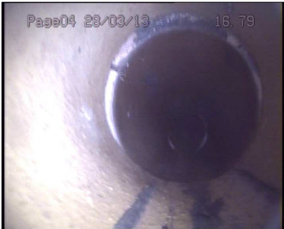
Photo: 1_1_26_A.jpg 16.8m, Joint displaced, medium (between 1.0 and 1.5 times the pipe wall thickness)
