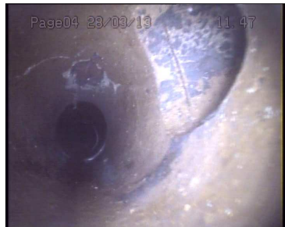
Photo: 1_1_17_A.jpg 11.5m, Connection, at 3 o'clock, 100mm diameter
